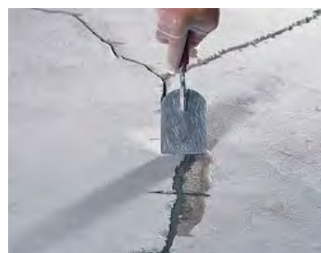
Crack needling with screed-clamps No. 75
