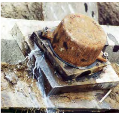
Anchor head during injection with HydroStop AcriGel 730 / HydroStop AcriBlend 740
