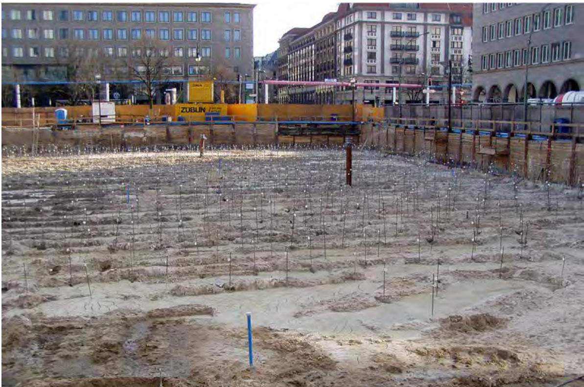
Bottom sealing with PurSeal SI 911 & AquaSoil 717 Integra
